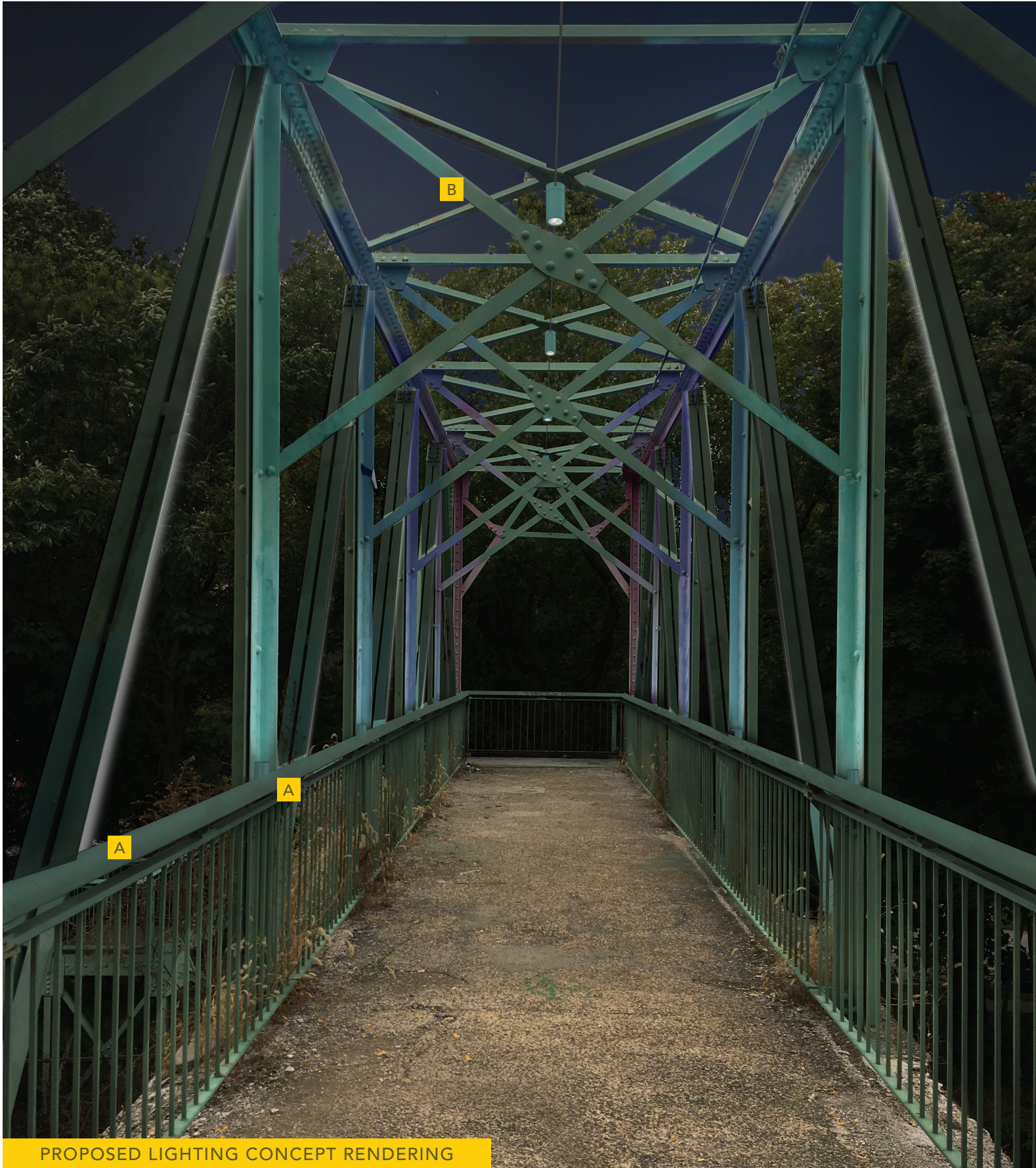
A COLOR-CHANGING LED UPLIGHT AT VERTICAL AND DIAGONAL MEMBERS CONCEALED BEHIND RAILING
